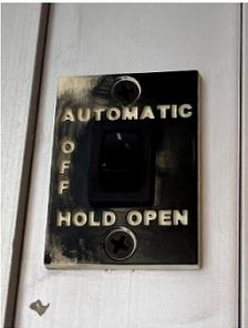
You may be aware that our handicap door sometimes has issues and refuses to open. The toggle switch at the top of the door should be in the “AUTOMATIC” position. If it is and the door is still not working, make sure you are pressing firmly in the center of the button, especially outside. Sometimes it just takes an extra bit of “oomph” to get it to work.
